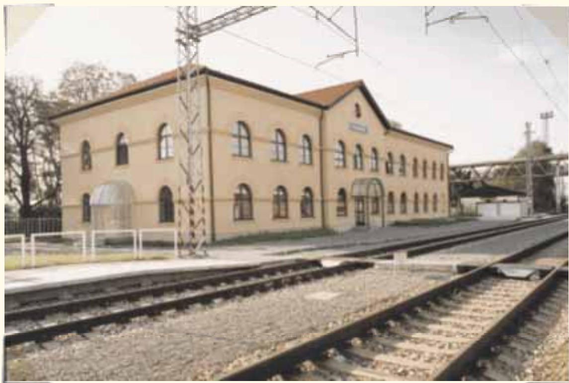
Modernizace trati Hodonín-Břeclav, žel. stanice Hodonín Modernization of Hodonín-Břeclav railway track, Hodonín railway station
