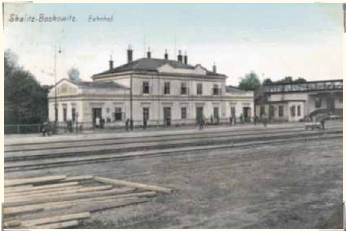
Žel. stanice Skalice nad Svitavou (1905-1914) Skalice nad Svitavou railway station (1905-1914)
