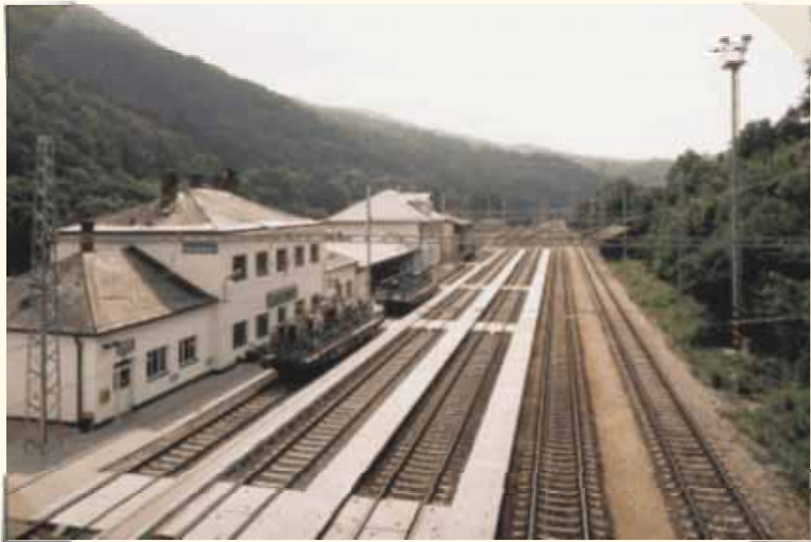
Optimalizace trati Brno-Skalice nad Svitavou, žel. stanice Adamov Optimising of Brno-Skalice nad Svitavou railway track, Adamov railway station
